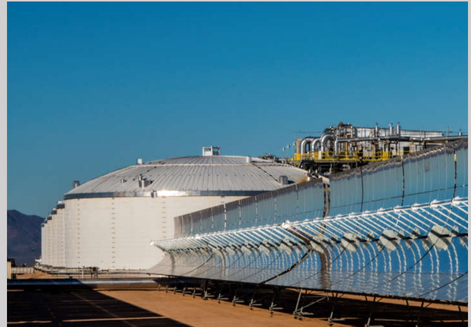
250-MW Solana Generating Station (Arizona, USA) with 6 hours of molten-salt thermal energy storage
