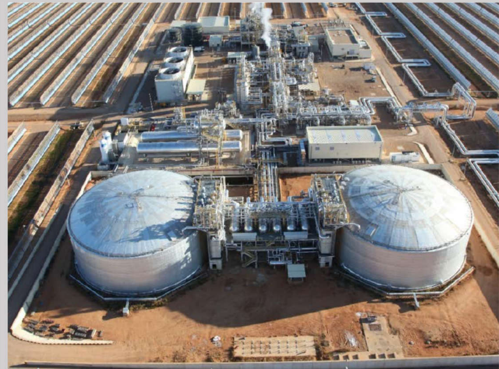
50-MW Termosol 1 Plant (Spain) with 9 hours of molten-salt TES
